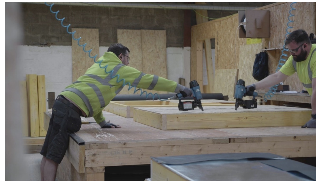
Constructing a timber kit
